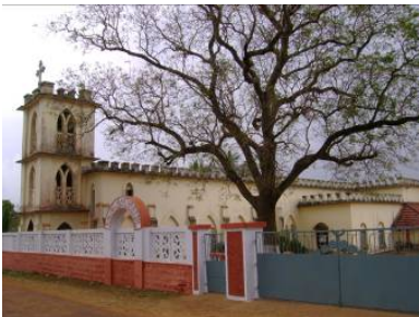
Fig. 11.34: A well preserved Church at Jatani
