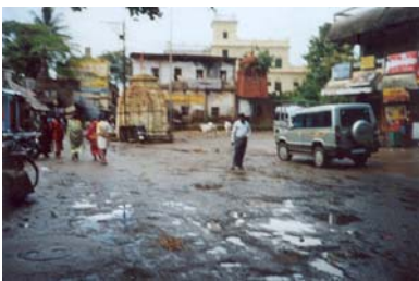
Fig. 11.29: Need for improvement of roads in the core heritage area
