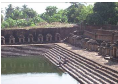
Fig. 11.11: A neglected tank
